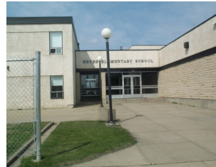
Main entrance at Heyes School. All guests to the school use this door.
